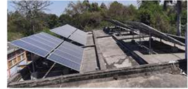
Installed 40 KWp at ITI Building Faizabad Railway station
